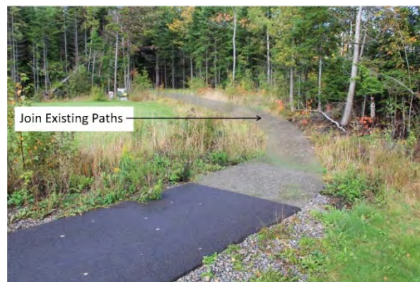
Completion of link between two existing paths in Oromocto West
